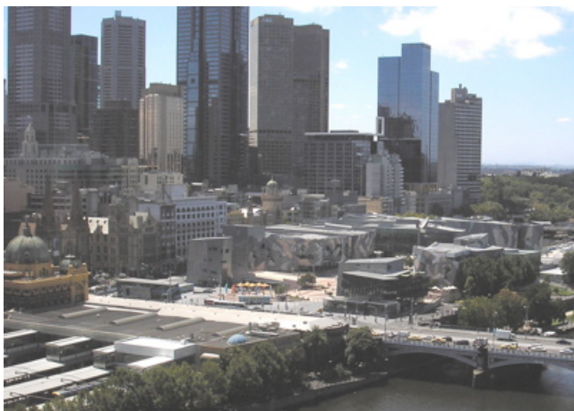
Figure 1: Federation Square, Melbourne, Australia
